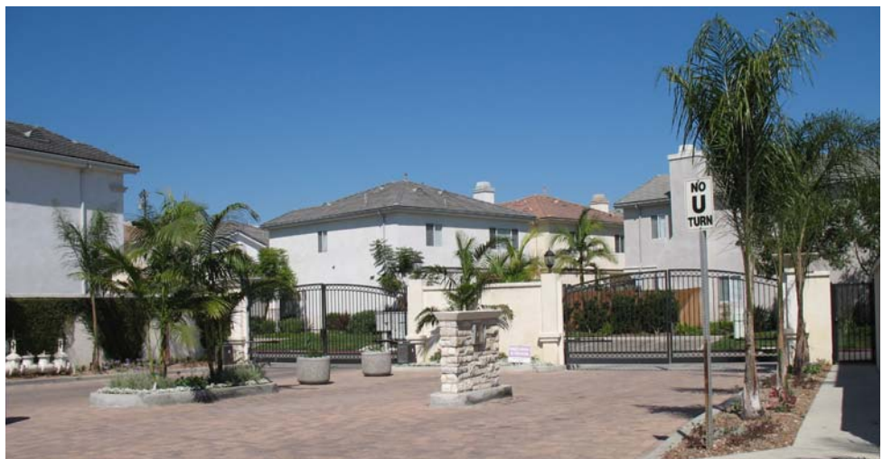
Graceful palms line the main entry, giving it the ambience of a tropical resort.
